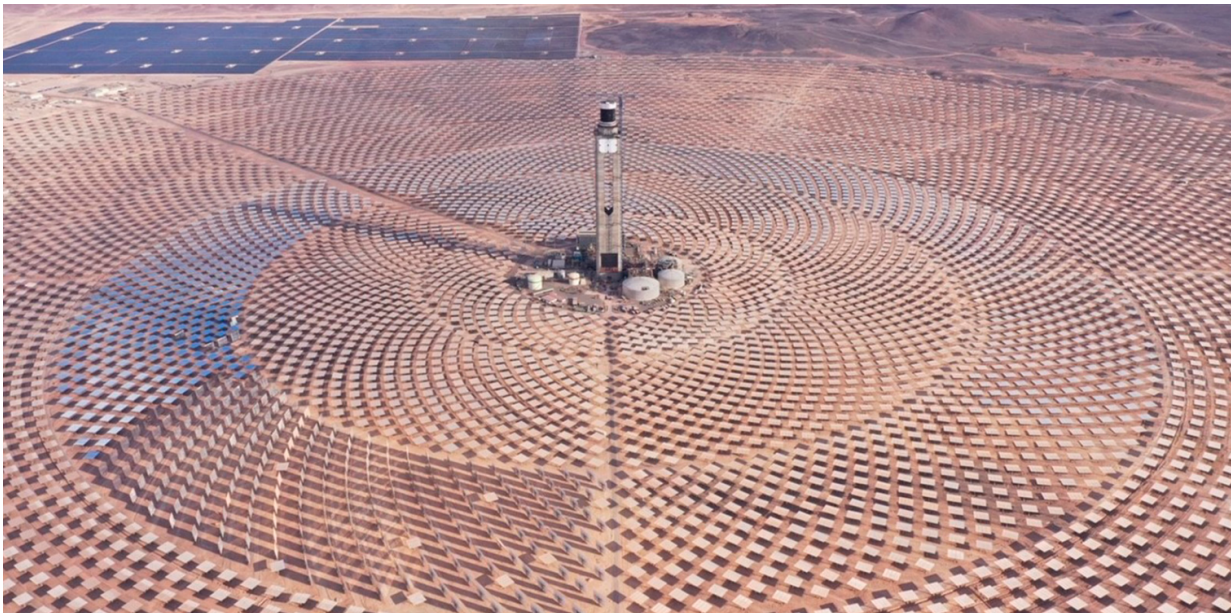
Figure 1.3: Dominador, a hybrid PV-CSP solar park in Chile (photo credit: [6])
