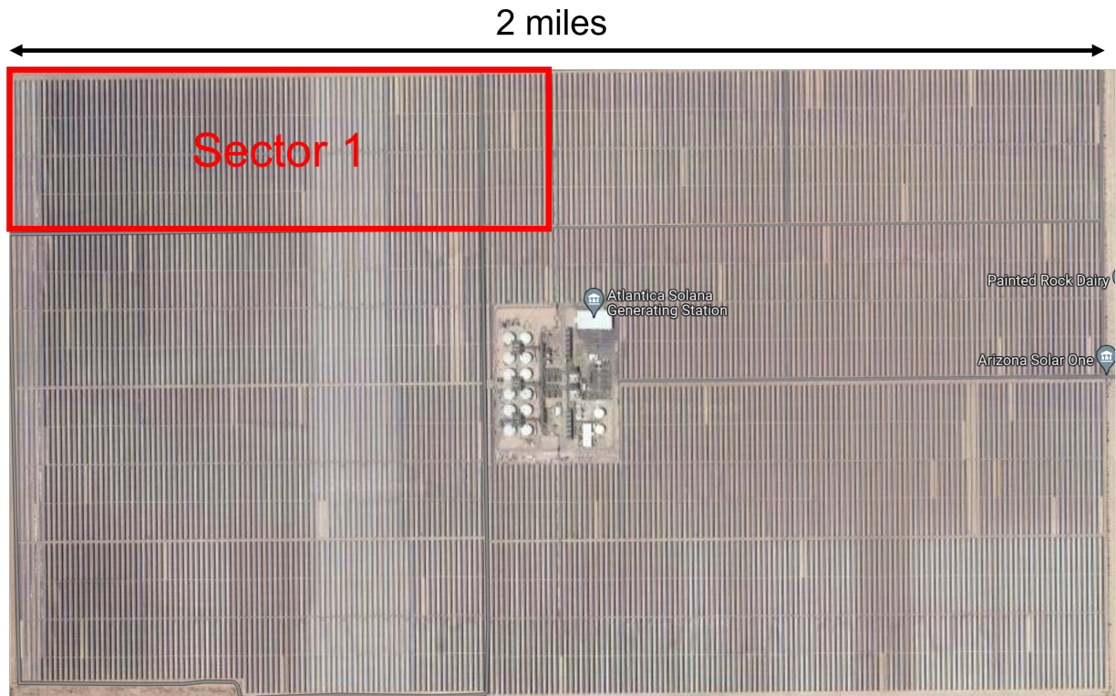
Figure 1.4: Google satellite image of Solana outlining one of eight sectors
